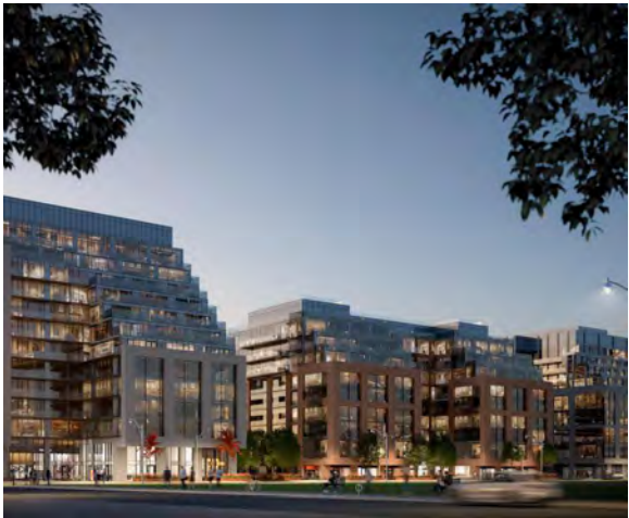
430-444 Dufferin Street 13 Storeys Under Construction
