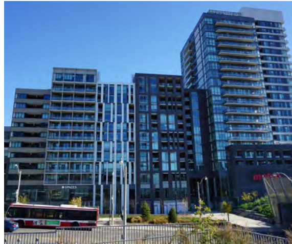
Figure 6: Development at 11 Peel Avenue
