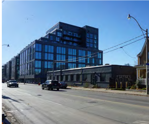
Figure 2: Legal Non-Conforming Townhomes, 450 Dufferin, and The Brixton Looking South on Dufferin Street
