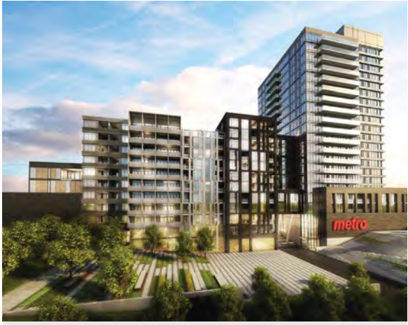
11 Peel Avenue 20 Storeys Built
