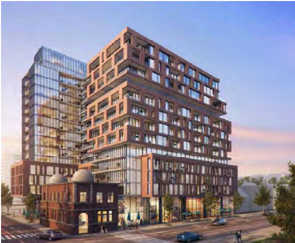
1221 King Street West 14 Storeys Under Construction
