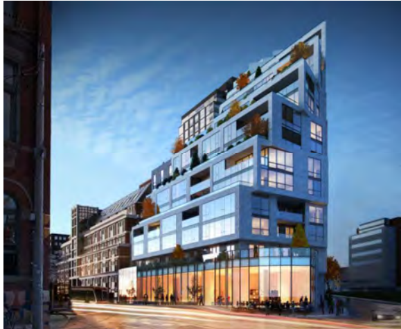
1181 Queen Street West 15 Storeys Under Construction
