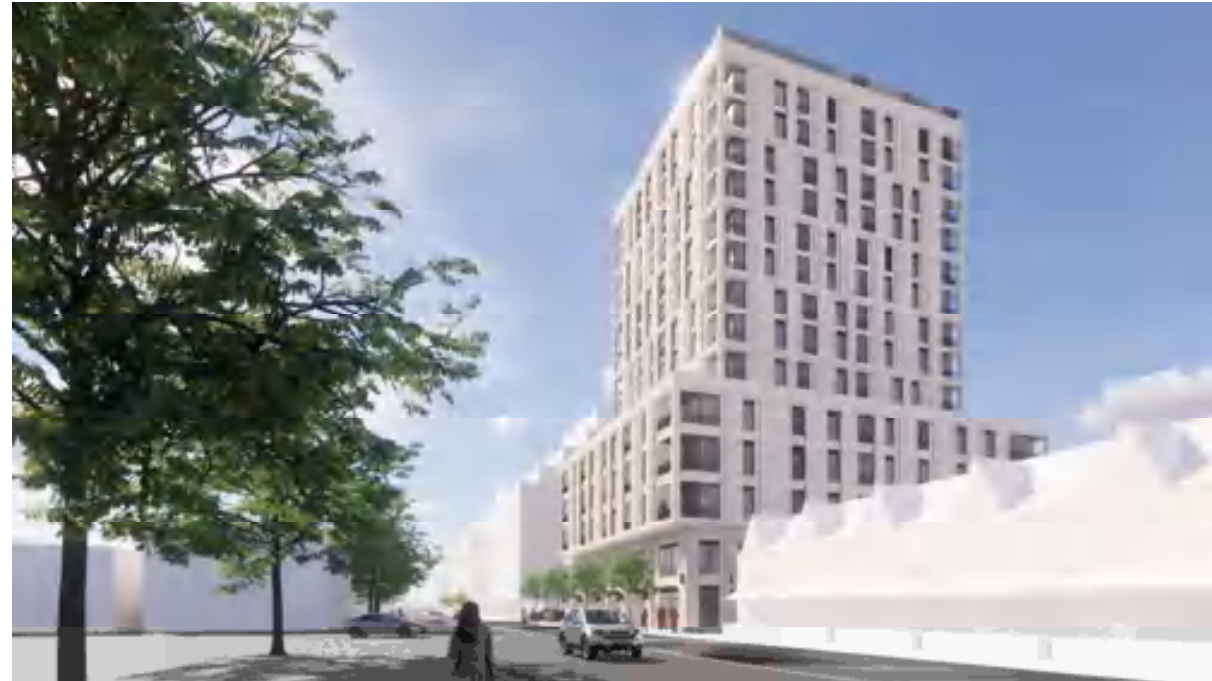
VIEW FROM DUFFERIN LOOKING SOUTH-WEST
